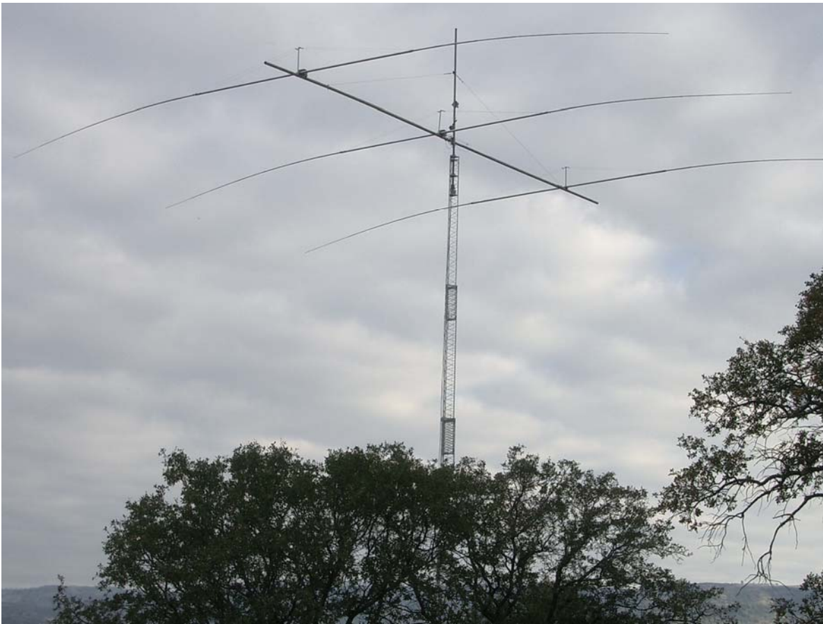
The 80M3LLA at K6MYC, North of Fresno CA. Tower is a US TOWER, 589 HDX with special 3" mast provision. Rotator is the OR2800 with 400 feet of control line. Note the 72' boom ready for the later expansion to 71' between the elements.
